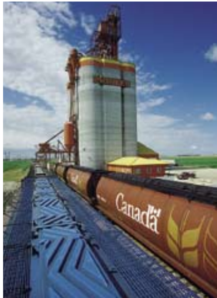
One of the new concrete elevators (silos) that are replacing the traditional wooden structures. In Western Canada, wheat and barley for export and domestic food use are marketed by the Canadian Wheat Board, a farmer-financed marketing agency with a government-granted monopoly. But elevators (silos) and other facilities are operated by private companies, which also market other crops for export and domestic sales.
