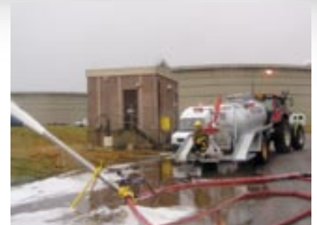
Water from the high pressure mains may be piped through the monitor on the rear of the tanker or the foam chemical can be piped to free standing monitors as here.
